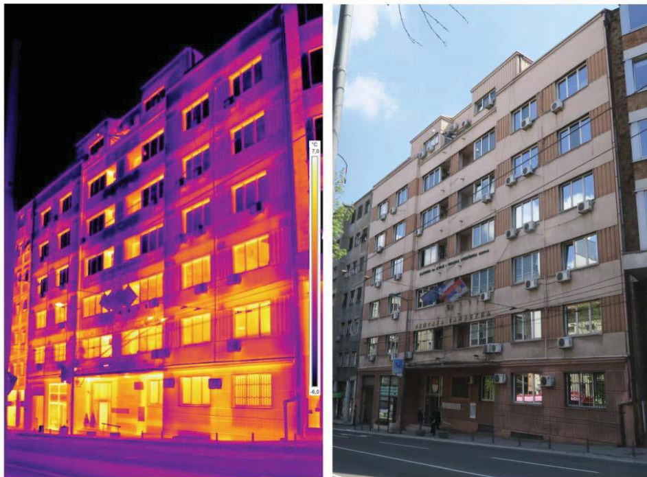
Figure 1. Thermal imaging and photograph of the street facade of the building of the City Municipality of Palilula. The image clearly shows heat losses in horizontal reinforced concrete elements as well as the beams over windows. No vertical reinforced concrete elements are observed
